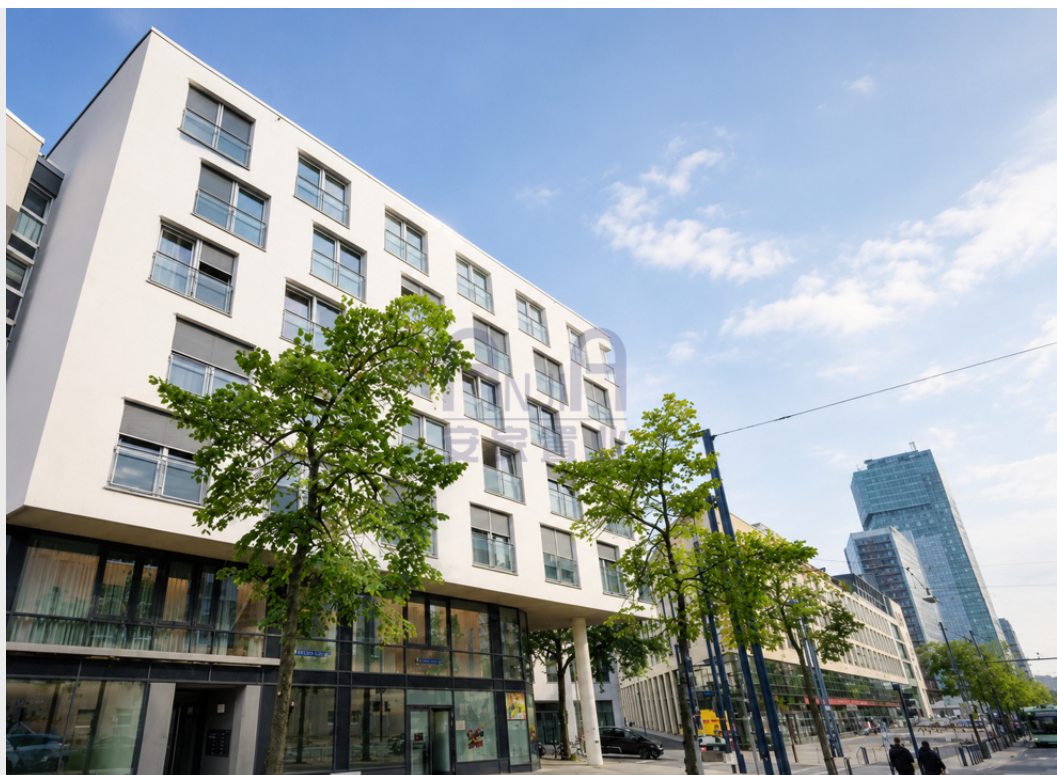
Berliner Strasse 34, 63065 Offenbach am Main, Germany
