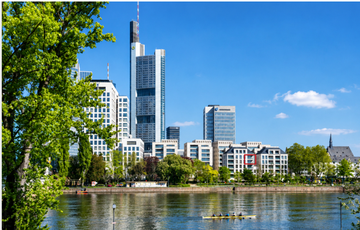
60311 Frankfurt am Main / Altstadt, Germany
